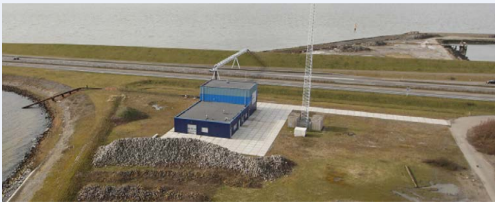
Fig.2 Full scale 50 kW RED research facility at the Afsluitdijk in the North of The Netherlands [1].
