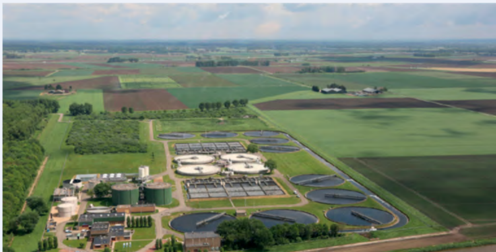
Fig 1. Municipal wastewater treatment plant BATH. This WWTP treats wastewater for 500,000 person equivalents and has the potential to supply biomass to produce 2000-2500 ton PHA/year [1] .
