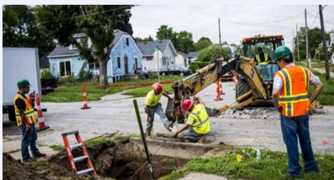
Figure 1: Water mains replacement
