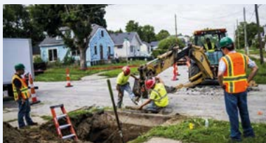
Figure 1: Water mains replacement
