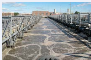
Fig.1. Sludge in the aeration basin of a WWTP
