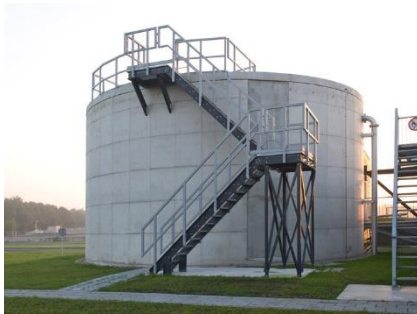
Figure 1 – Full-scale BODAC filter at Puurwater Fabriek, Emmen, The Netherlands 2 .
