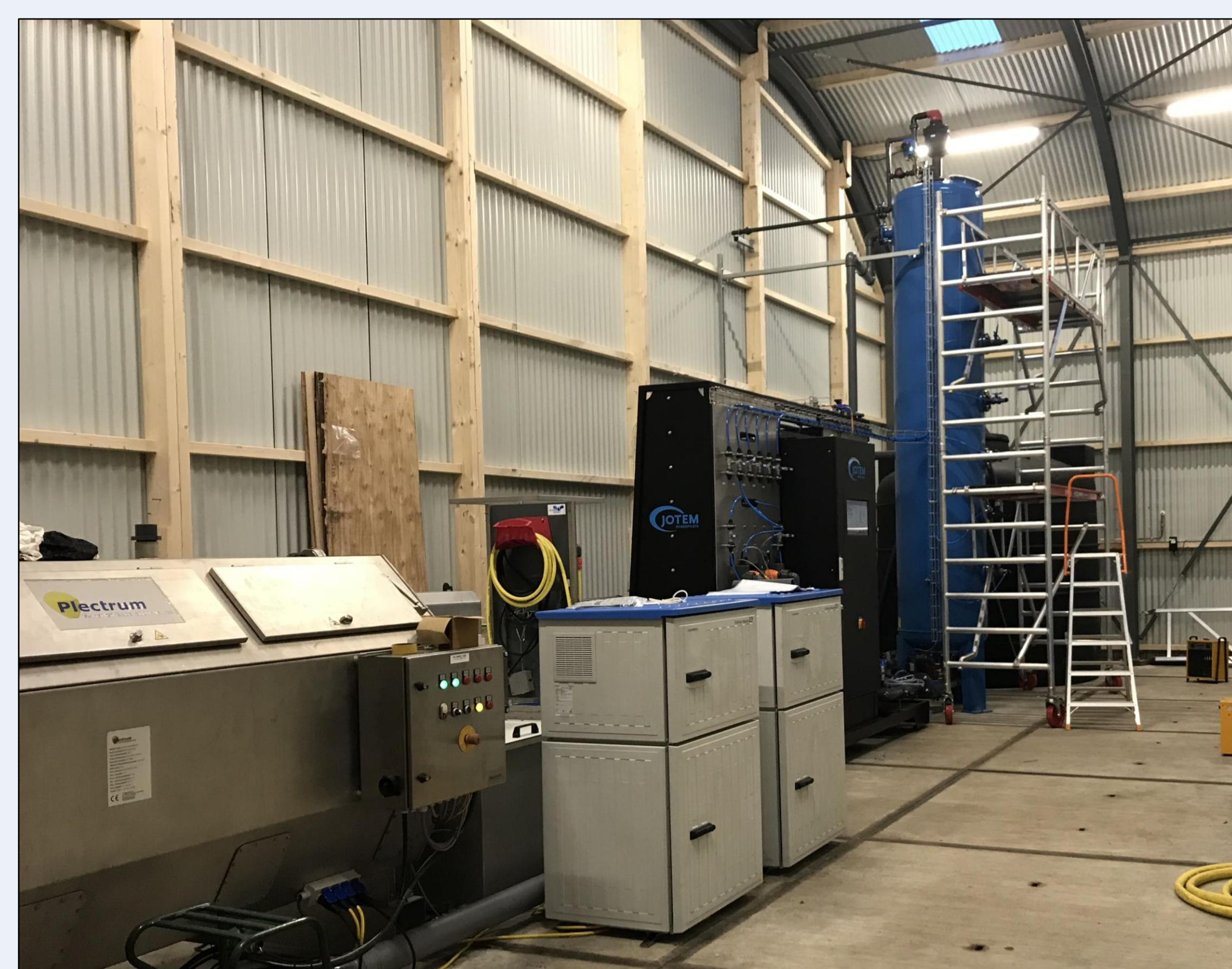
Fig. 1 Pilot installation of the BODAC filter
