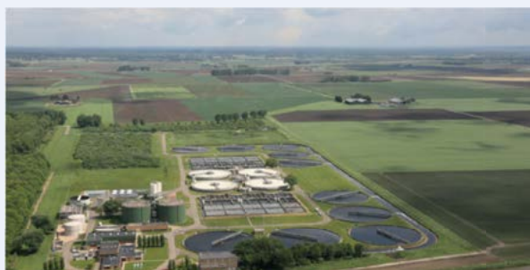
Fig 1. Municipal wastewater treatment plant BATH. This WWTP treats wastewater for 500,000 person equivalents and has the potential to supply biomass to produce 2000-2500 ton PHA/year [1] .
