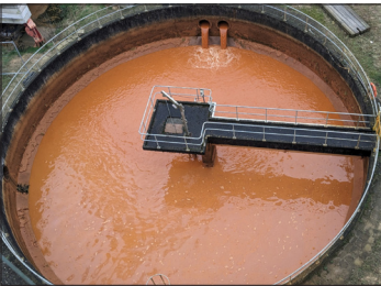
Iron sludge basin Aquafer is also available in pellet or granulate form. The iron is a suspension of ferric (hydr)oxide that results from the process of iron-removal from groundwater. The pellets/granulates are made by adding carboxymethyl cellulose (CMC), drying the sludge and then transforming it into pellets/granulates
